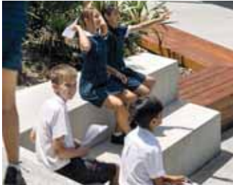
CONCRETE SEATING WALLS 350mm (H) x 600mm (D) Length varies Insitu off form concrete Colour: Portland grey
